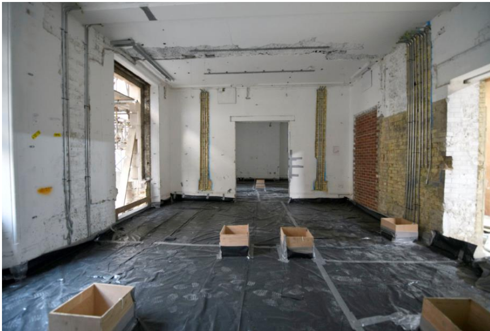
Residential Lobby builders works
