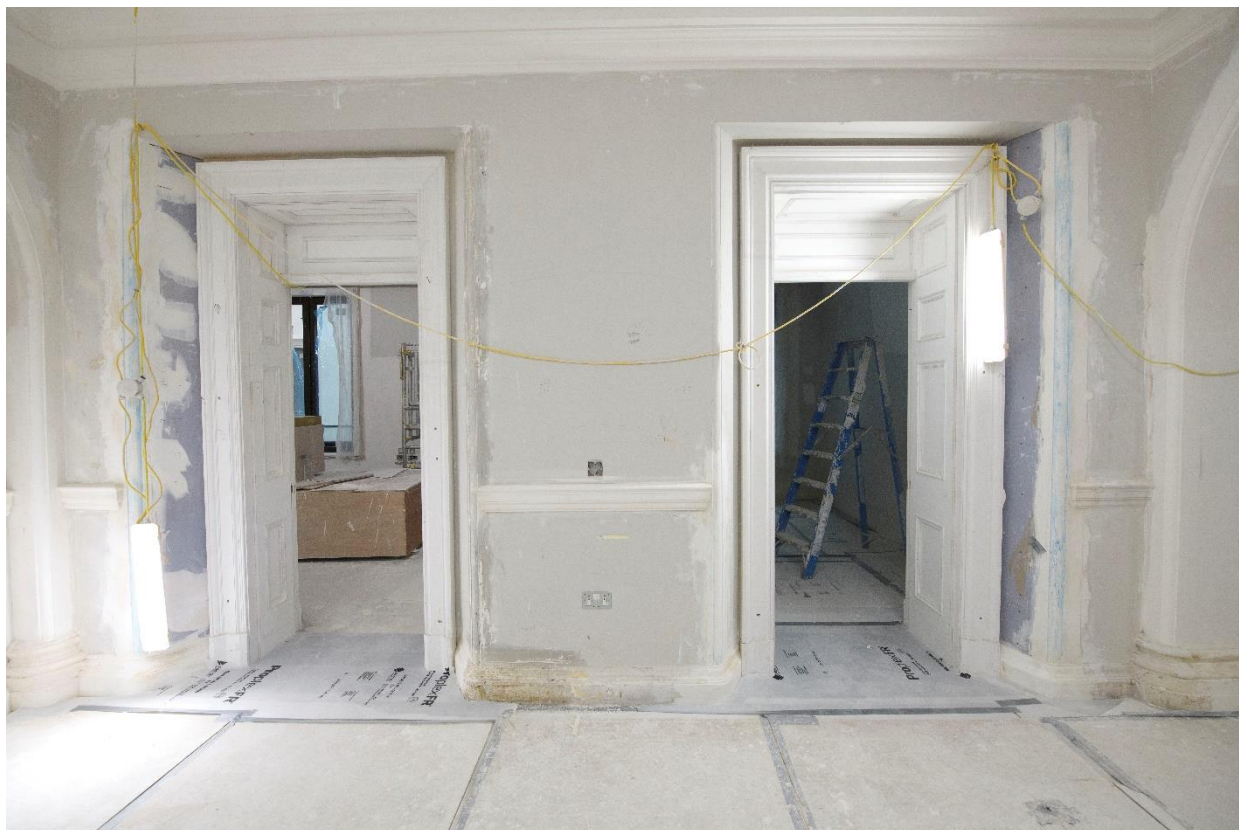
Level 3 Resi fitout
