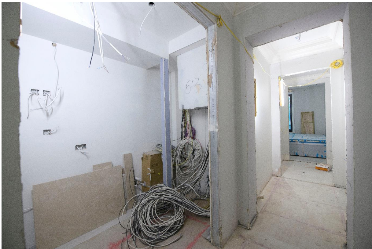
Level 4 Resi fitout
