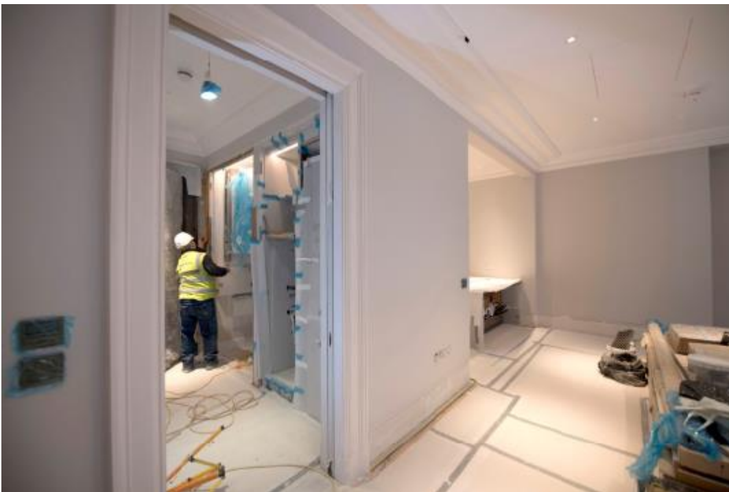
Level 3 Resi Fitout
