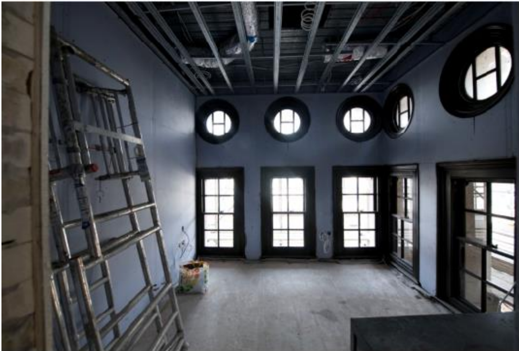
Level 6 Resi Fitout
