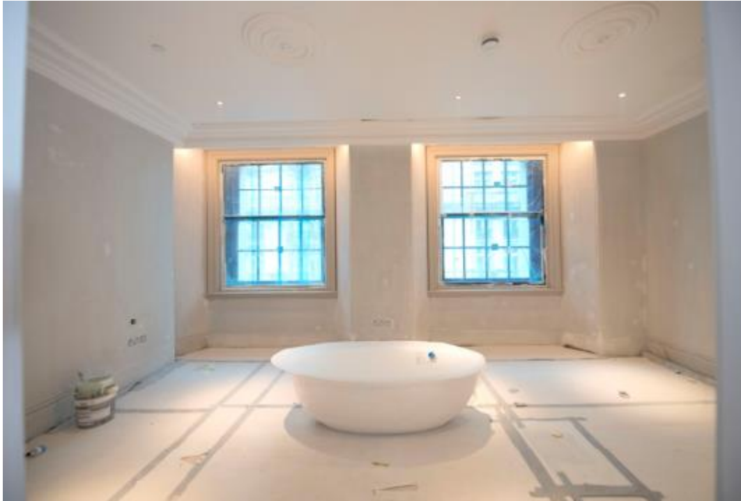
Level 4 Resi Fitout
