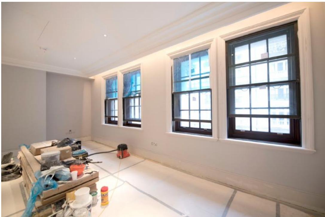
Level 3 Resi Fitout
