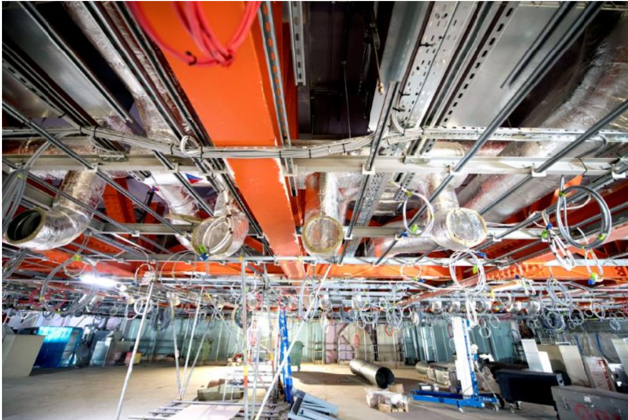
Basement 1 Ballroom ceiling
