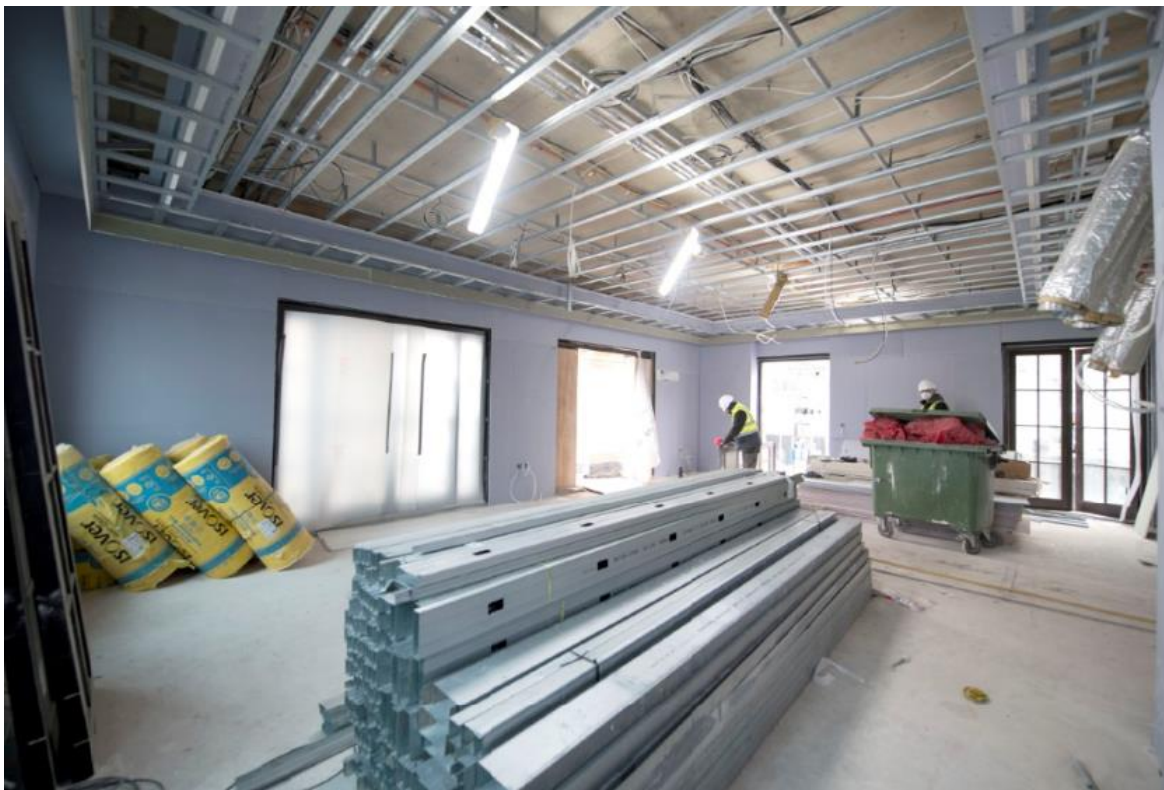
Level 7 Penthouse fitout
