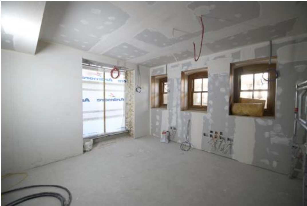
Level 5 Resi fitout
