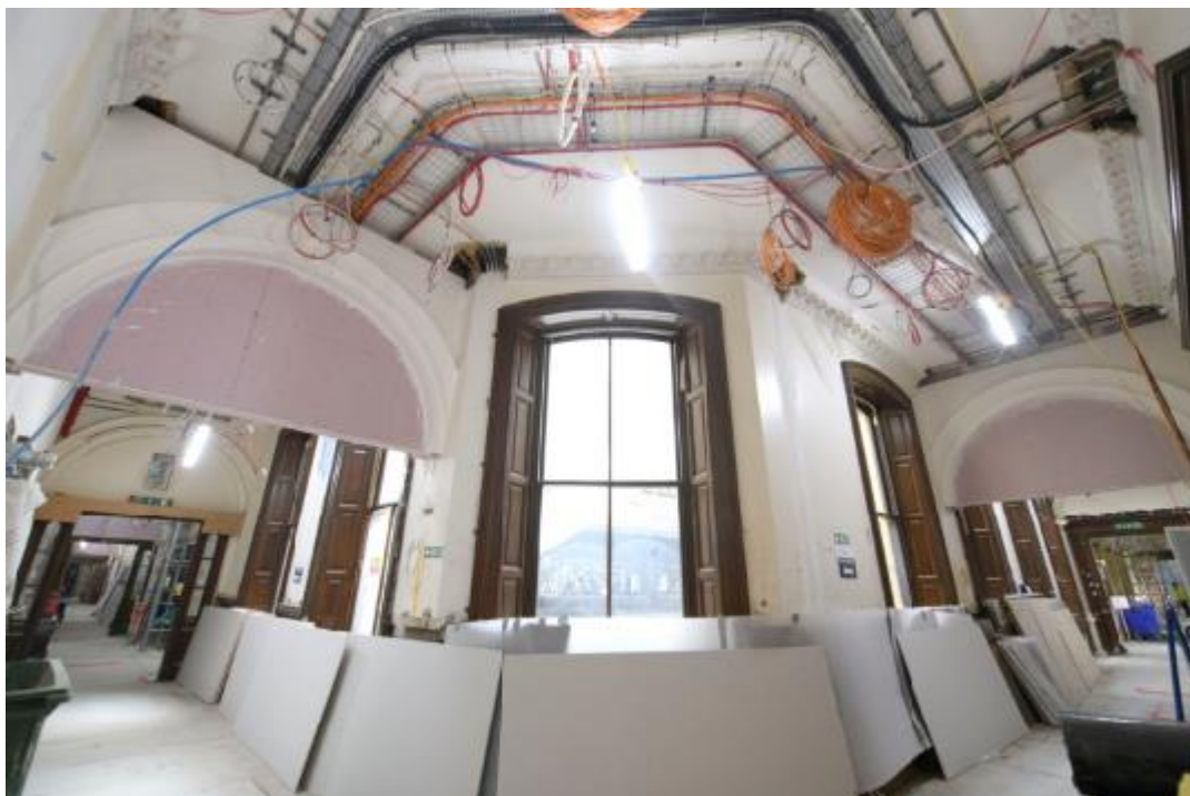
Level 2 Hotel Corridor
