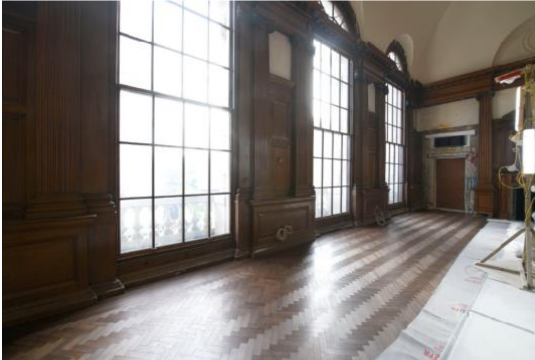
Level 2 Heritage room Fitout
