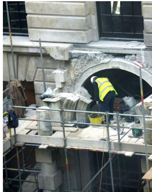
Ground floor quadrangle courtyard stone repair.
