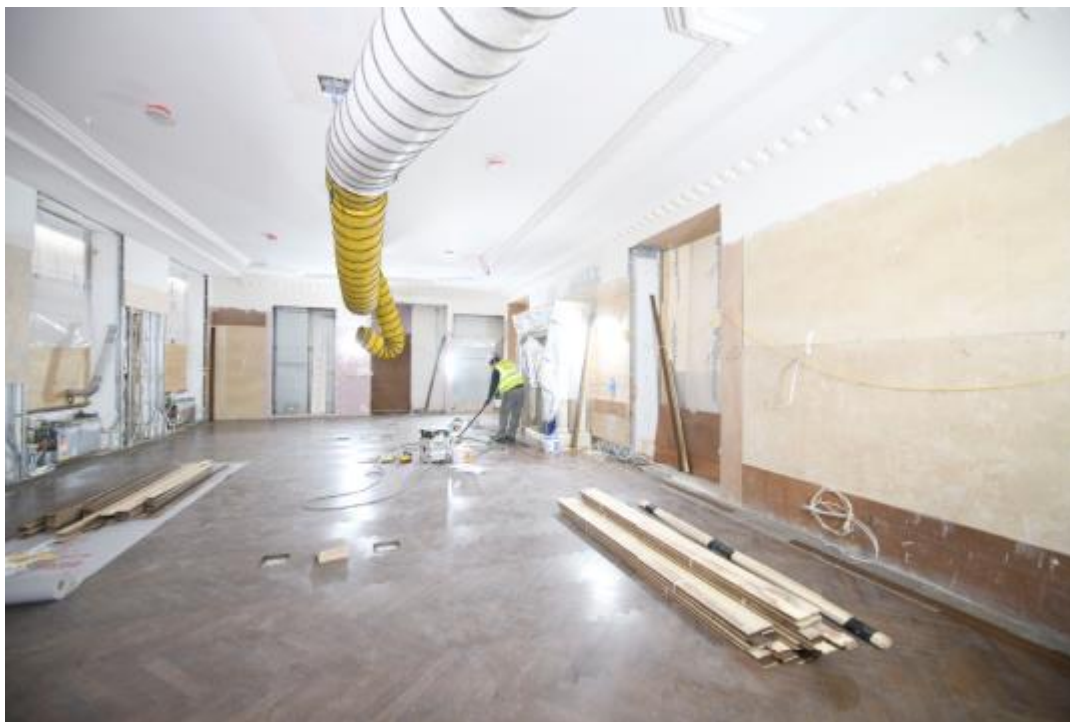
Ground Floor FoH fitout
