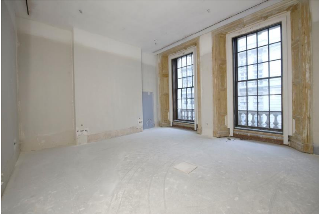
Level 2 resi Fitout
