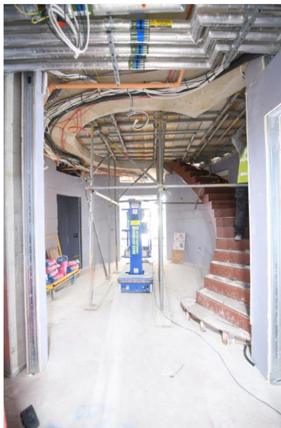
Level 6 Resi Fit out
