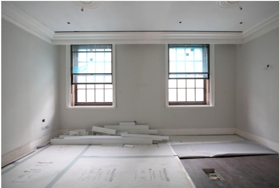
Level 3 Resi Fitout
