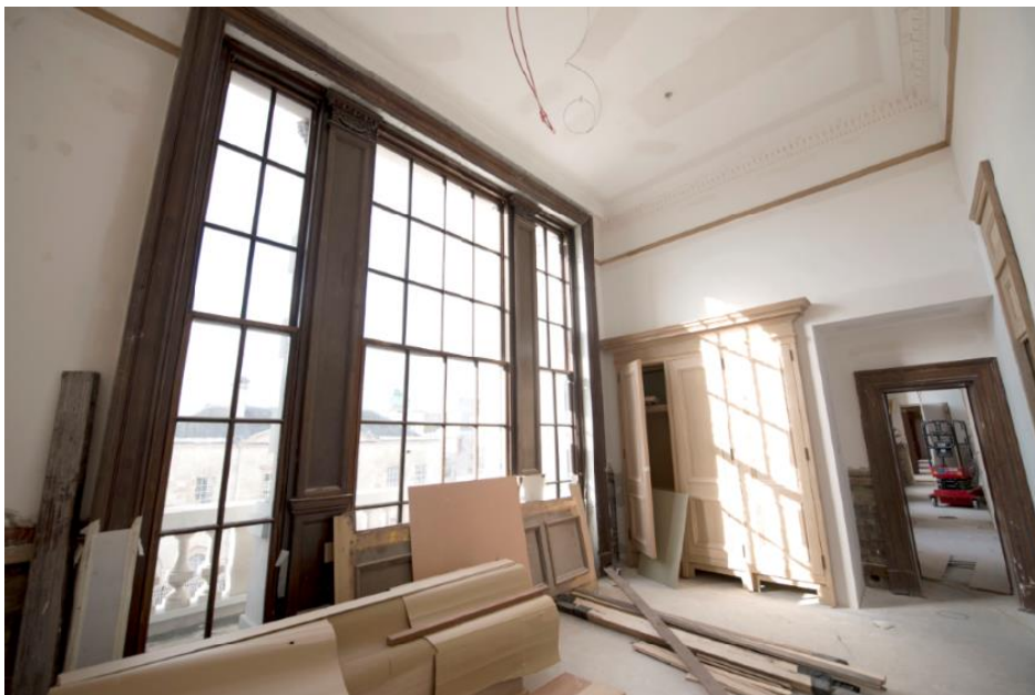
Level 2 Hotel Fitout
