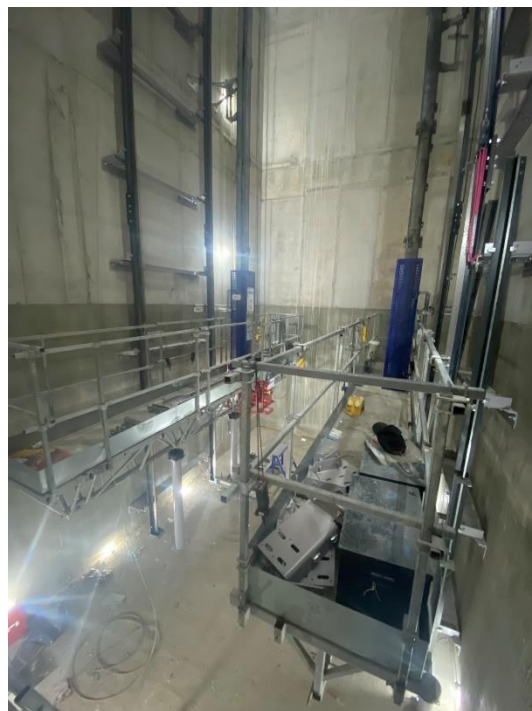
Basement 5 Car lift installation
