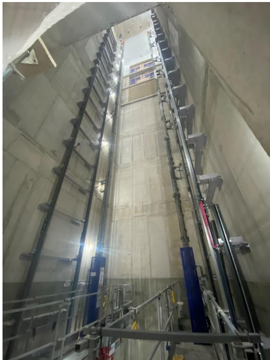
Basement 5 Car lift installation
