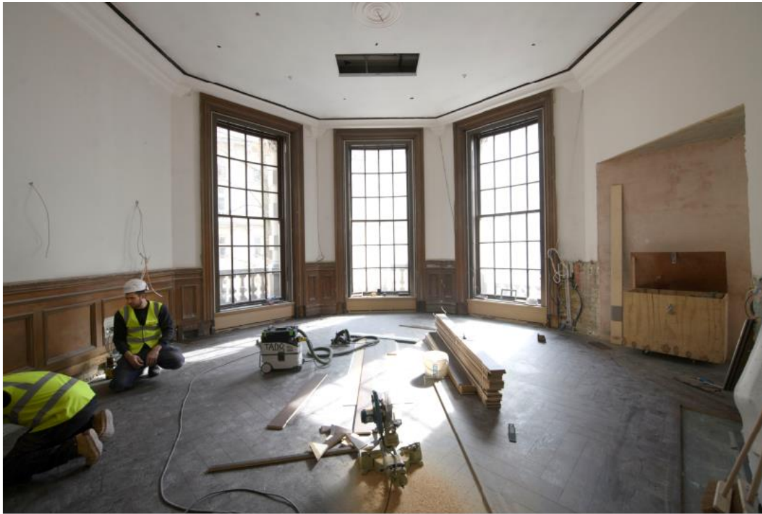
Level 2 Resi Fitout
