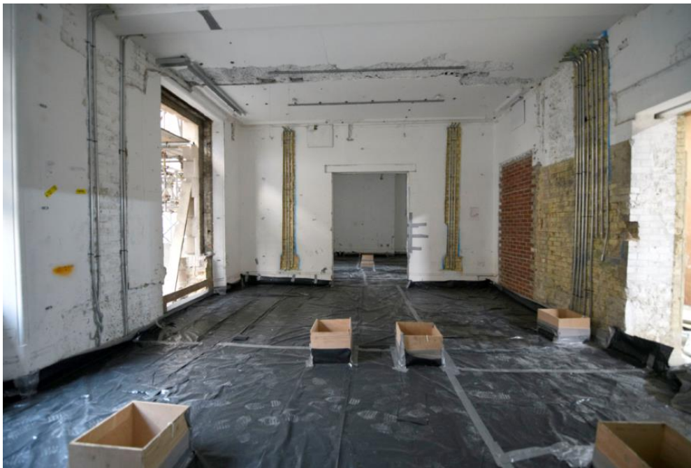
Residential Lobby builders works
