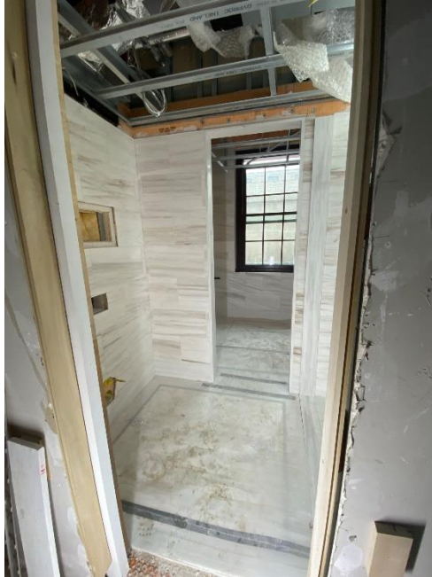
Hotel level 5 – hotel fitout
