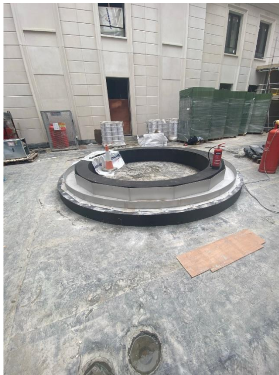
Triangular courtyard water feature.
