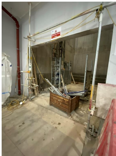
Basement 5 Hoist removal and lift works.
