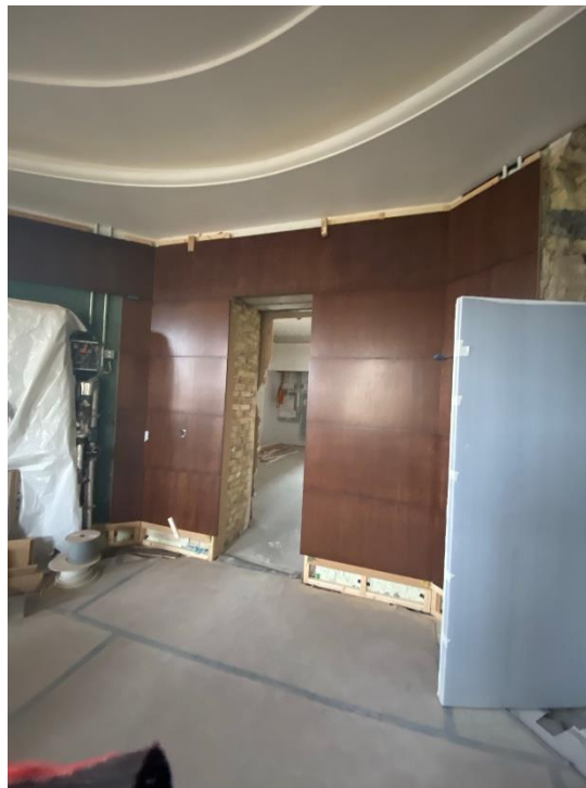
Level 3 Hotel fitout
