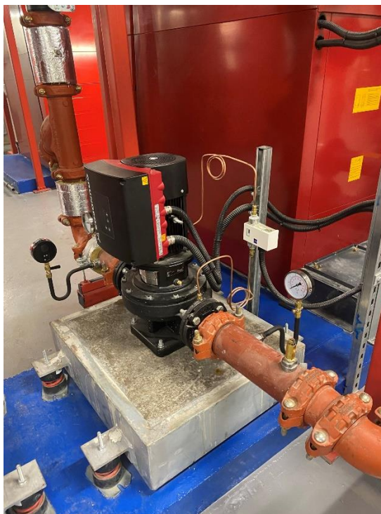
Basement 5 services installation
