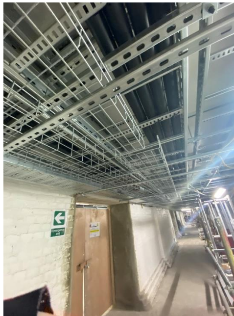
Basement 1 stair and LG services installation
