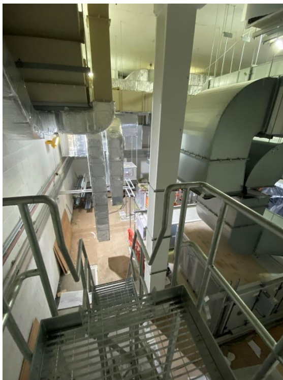
Basement 4 M&E installation plant room & Spa
