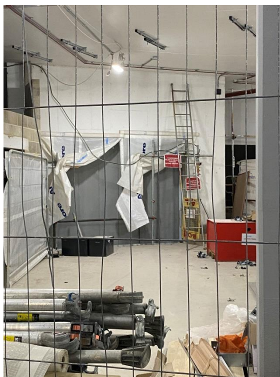
Basement 5 services installation
