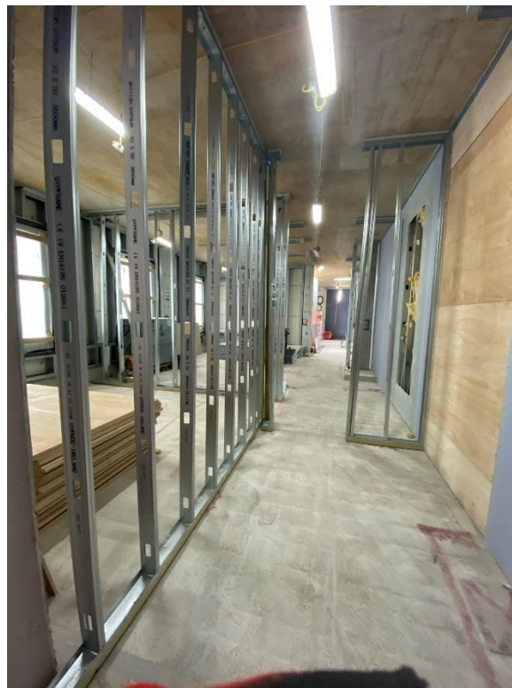
Level 5 Hotel and Residential Fitout
