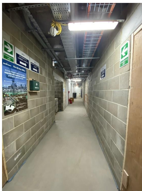
Basement 4 M&E installation plant room & Spa
