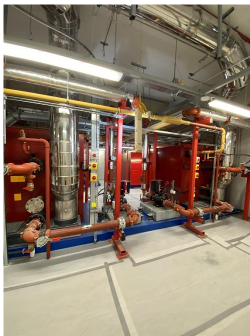
Basement 5 services installation
