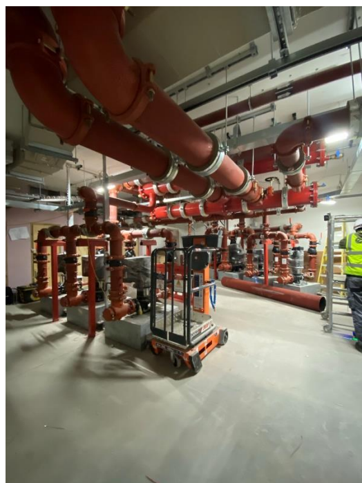
Basement 4 M&E installation plant room & Spa
