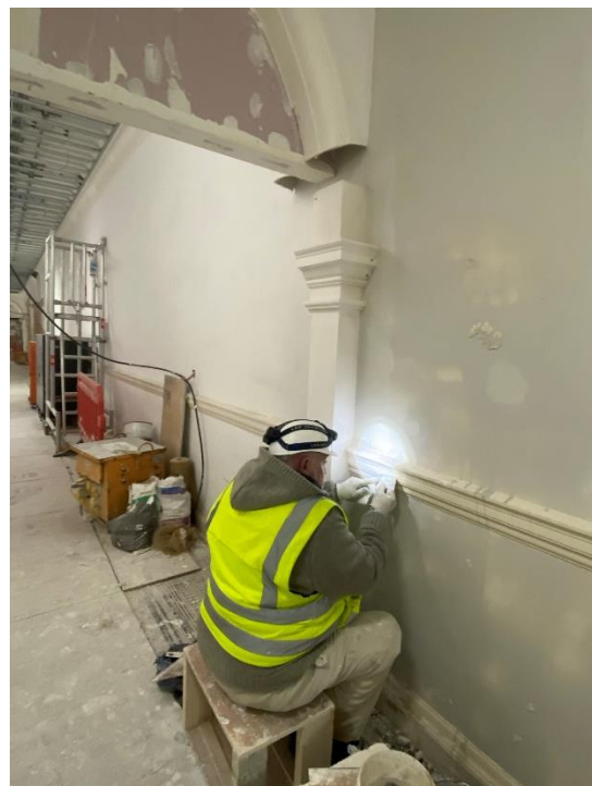
Level 3 Hotel Fitout
