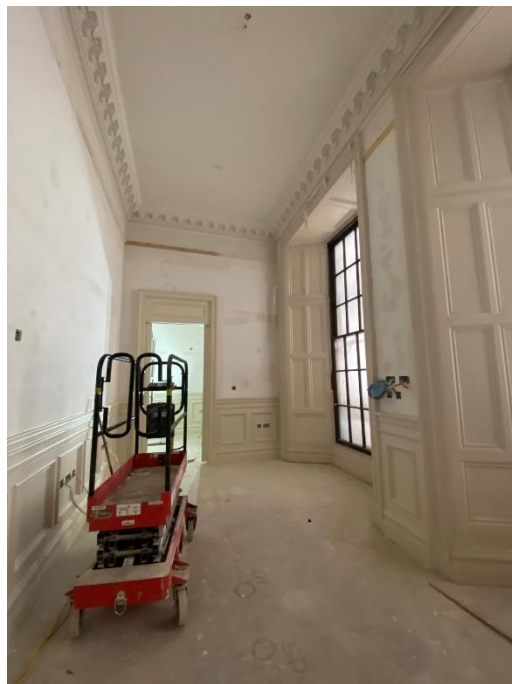
Level 2 Hotel Fitout
