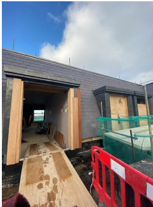
Level 7 Mansard roof
