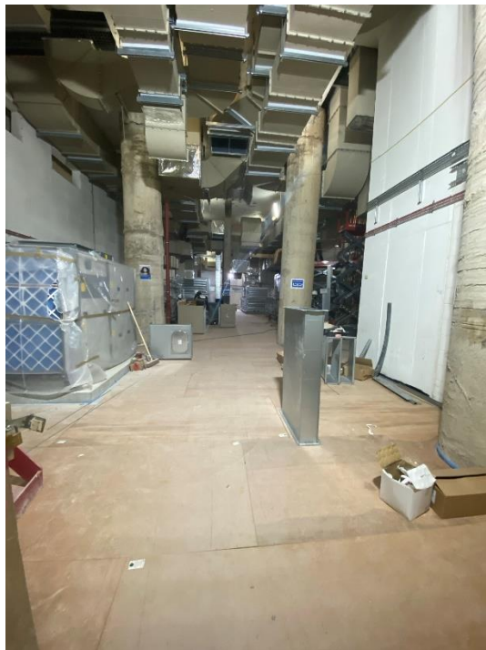
Basement 4 M&E installation plant room & Spa
