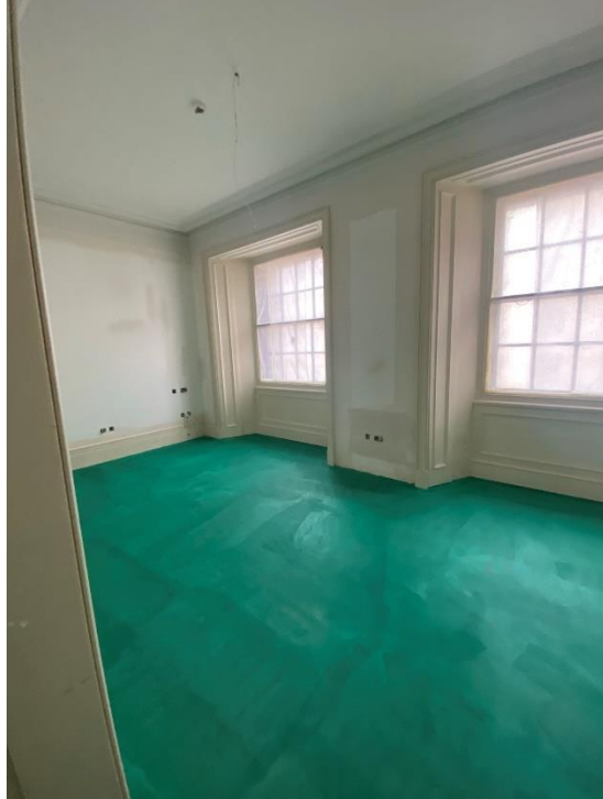
Level 3 Hotel Fitout
