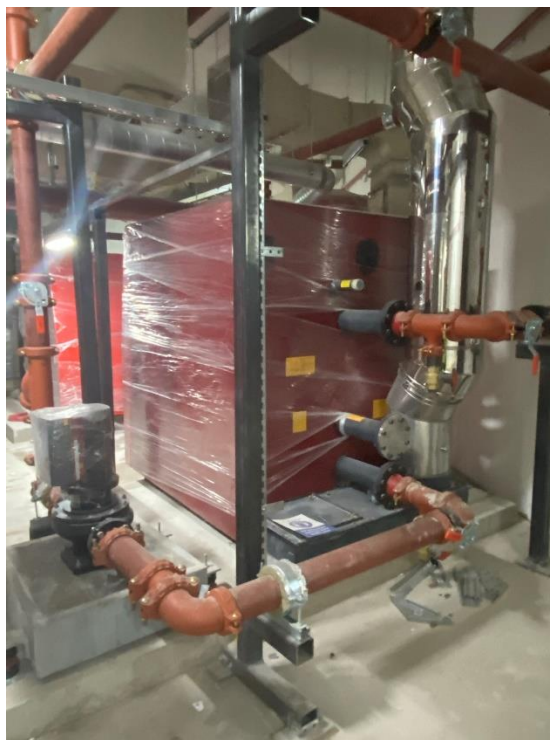
Basement 5 services installation.
