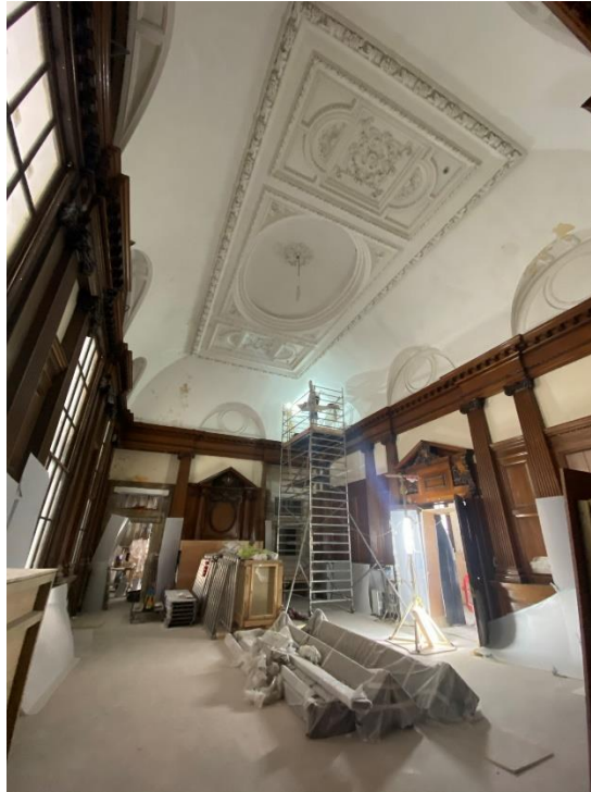
Level 2 Hotel Fitout
