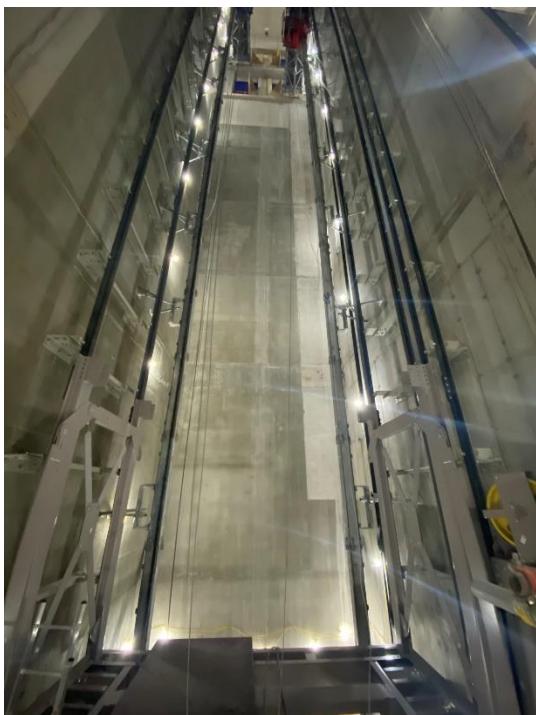
Basement 5 New Car Lift instalation
