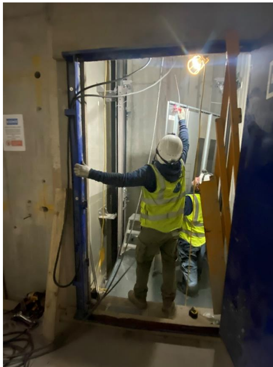
Basement 2 Insulation Lift Doors
