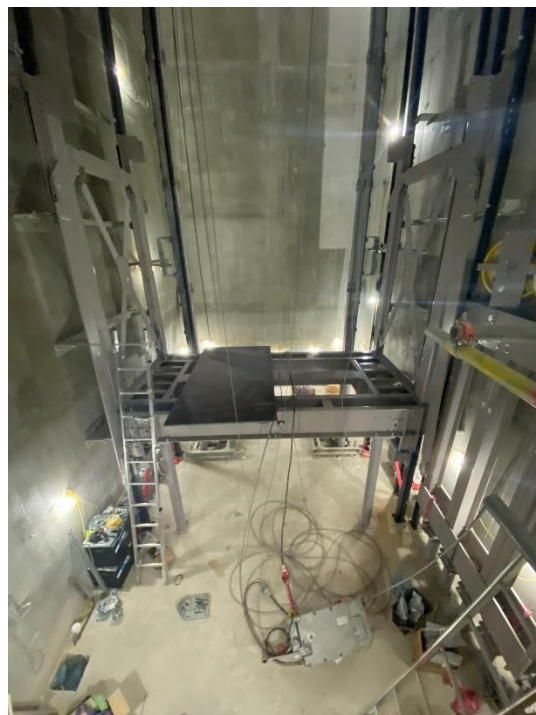
Basement 5 New Car Lift instalation
